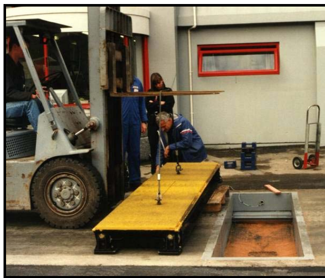
Figure 5.2.1.2 Typical construction of a fixed axle weighbridge
